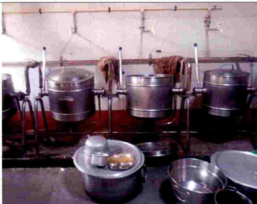
STEAM SYSTEM INSTALLED (FOR COOKING PURPOSE) IN HOSTEL KITCHEN.
